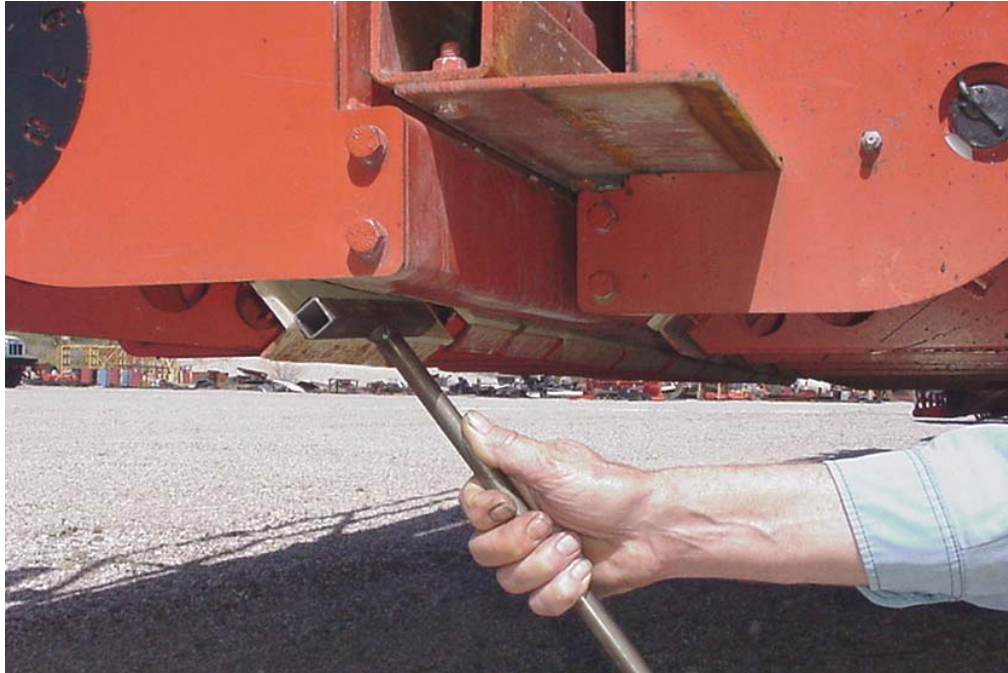
Figure 6-2. Checking Gate Opening
