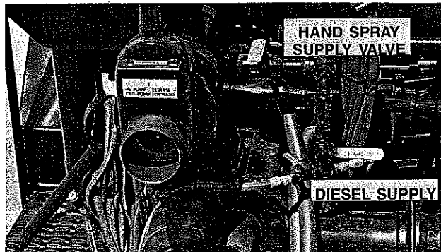
(4.1) HAND SPRAY & FLUSHING DIESEL SUPPLY VALVES
